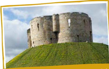
Flooding weakened the artificial mound and the tower's walls began to crack. Some parts of Clifford's Tower were close to collapse in the 1360s.
