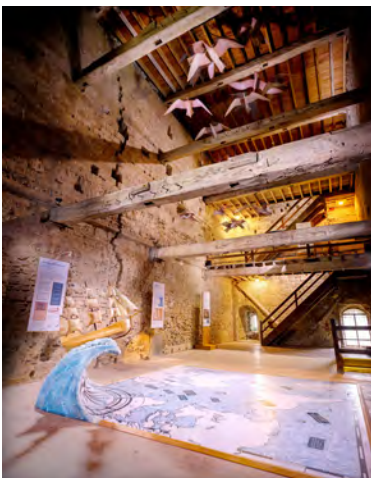
The second floor of the keep.
