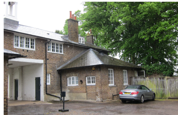
9. West (rear) elevation from yard
