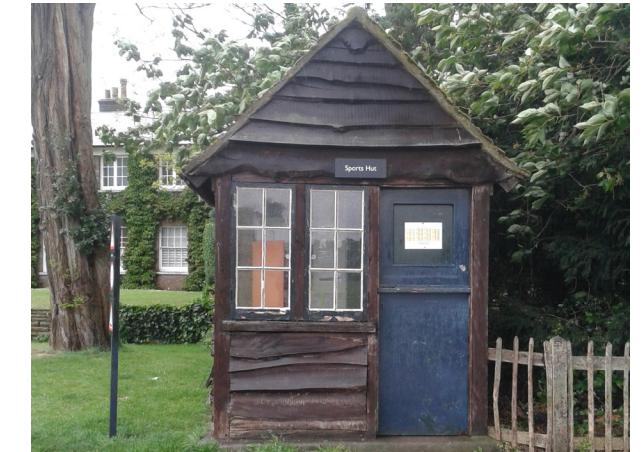
Ticket Machine Shed
