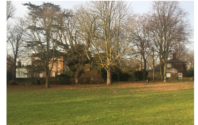
View of Southend House Boundary wall and Stable Block
