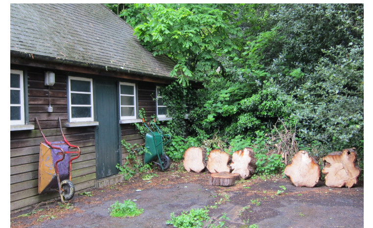
11. Former changing rooms to north of Stable Block
