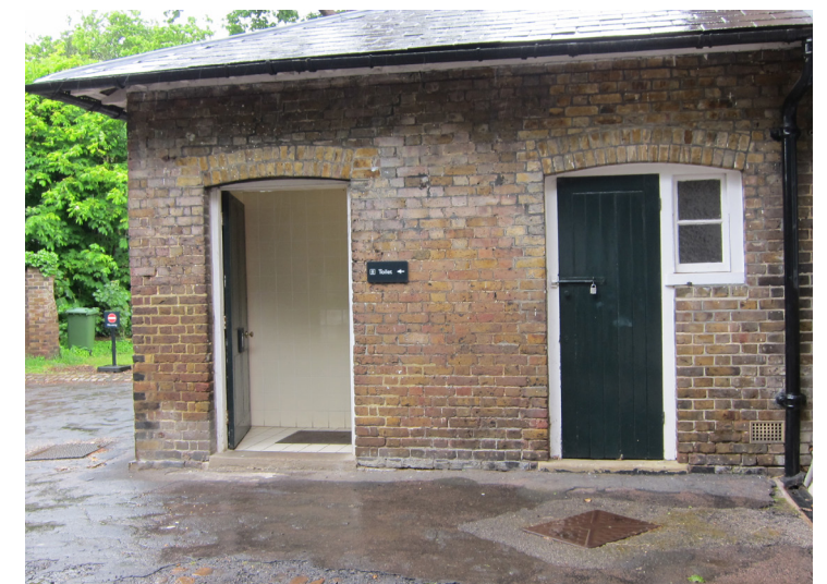
Existing Wc's to be upgraded
