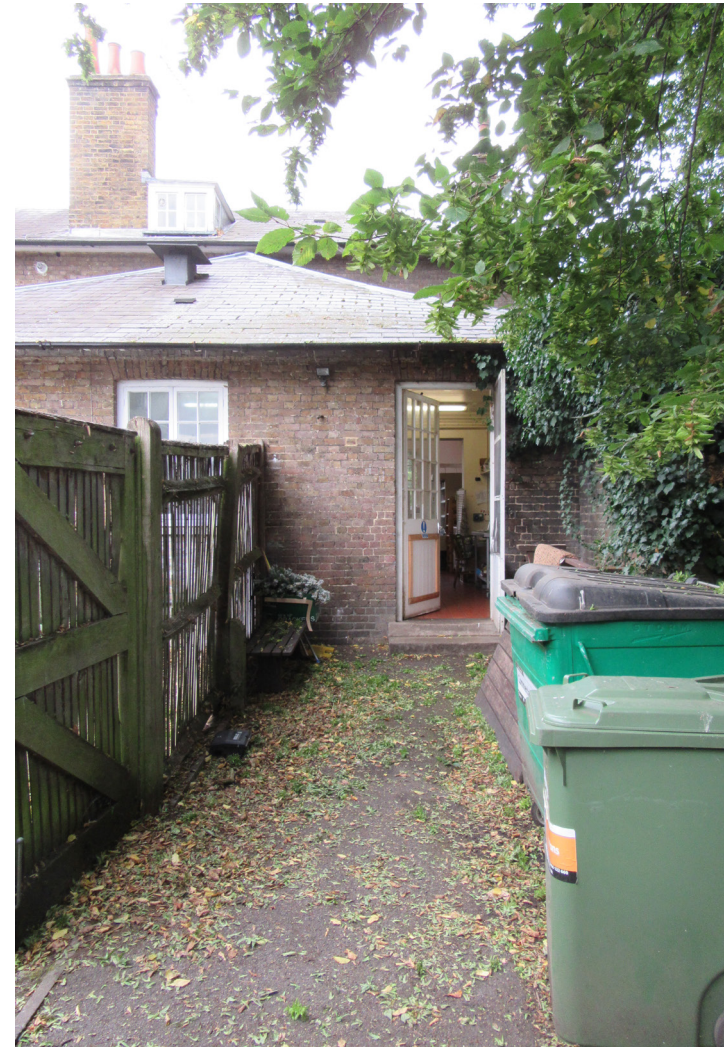
Existing bin store and kitchen door
