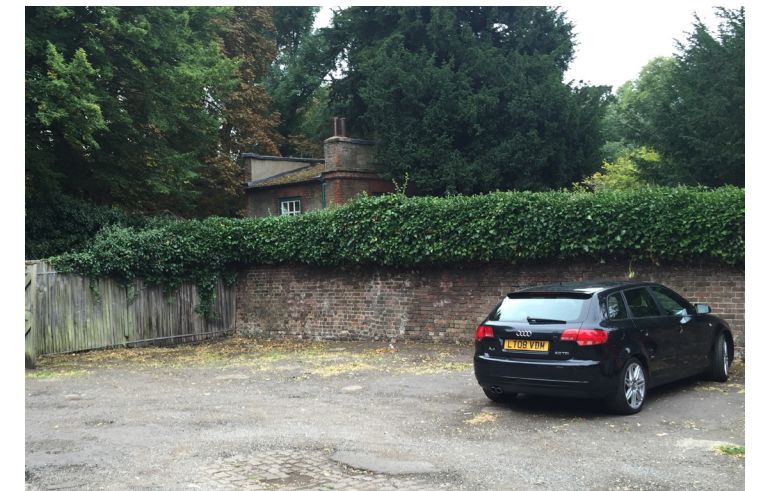
View of Boundary wall to Southend House from yard
