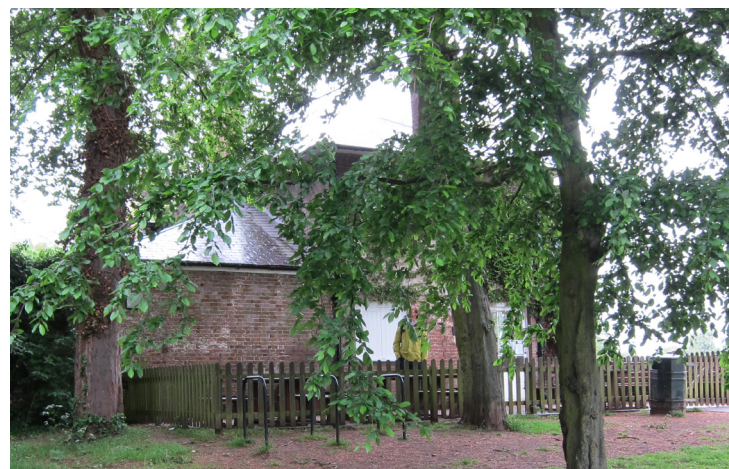
6. South elevation, boundary wall to yard. Ground falls away towards western meadow
