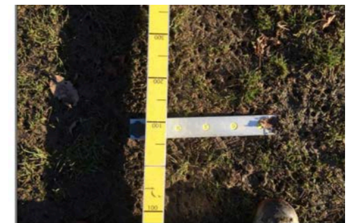
Plate 14: Undulation > 25mm depth – centre circle
