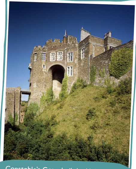
Constable's Gate, built by Hubert de Burgh in the early 13th century, rises from a huge battered (sloping) base from the bottom of the moat.
