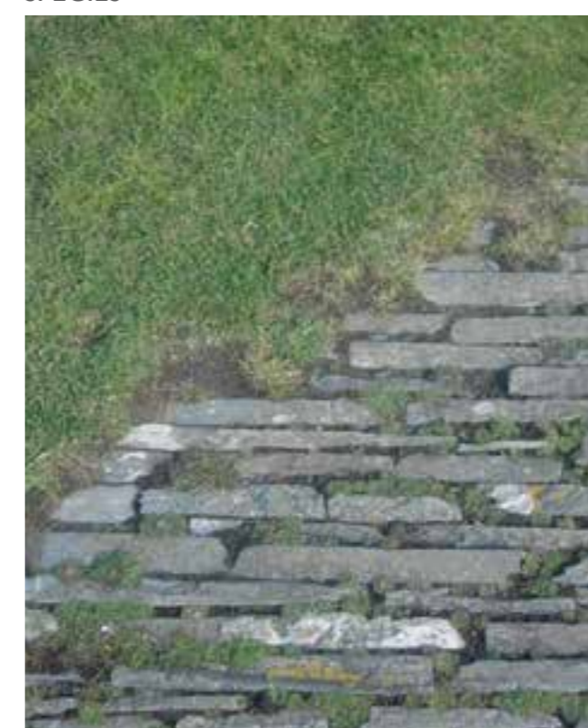
DELABOLE SLATE PITCHING USED IN HIGH FOOTFALL INTENSITY AREAS
