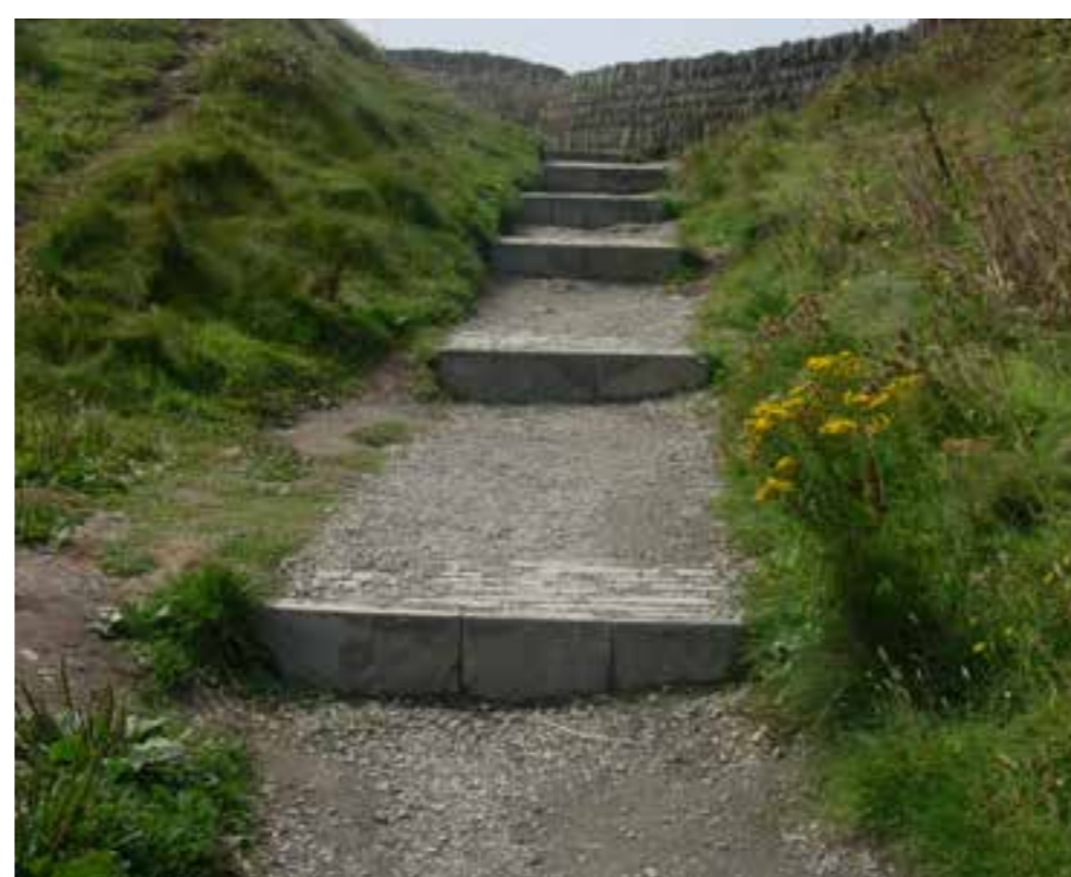
PROPOSED ACCESS PATH SURFACING AND STEPS TO MATCH SOME OF THE EXISTING
