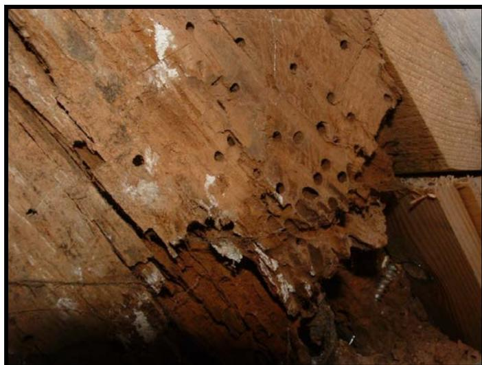
Ceiling timber has been attacked in this area because there has been water leakage from the roof above.
