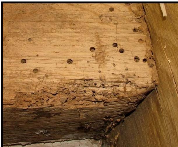
Fresh holes will have piles of bore dust, called frass, underneath
