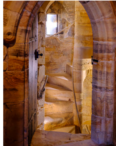
The gatehouse also has an exhibition, and you can admire views from the roof. It is accessed by steep narrow staircases like this.
