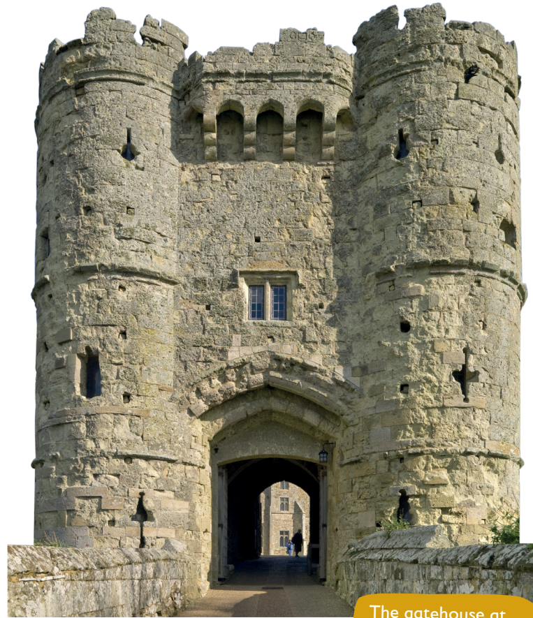
The gatehouse at Carisbrooke Castle.
