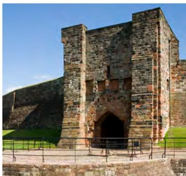
The buttresses supporting the Captain's Tower have chamfered bases to provide extra protection against battering and mining.
