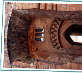
The brick archway above the windows in the Captain's Tower was added so the cannons could be transported over the top of the tower, along the walkway.
