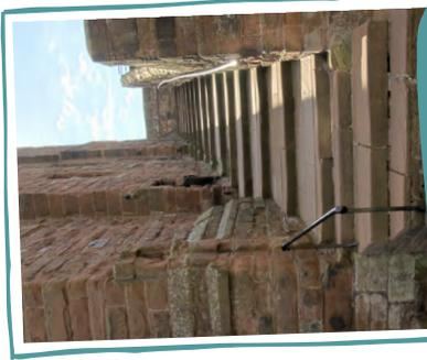
The steps used to be a ramp. It was built in the 16th century so that cannons could be pushed up to the walkway of the inner ward.
