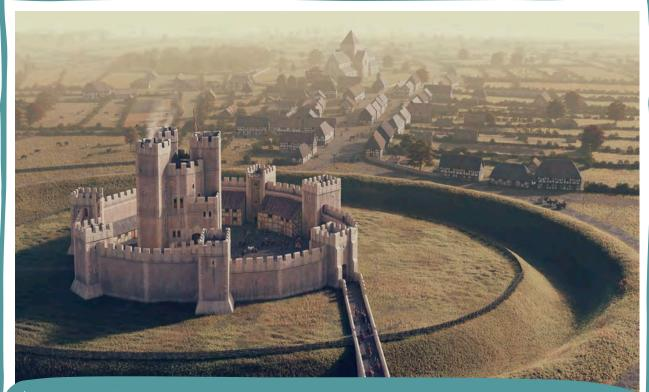
A reconstruction drawing showing Orford Castle from the south-east in the 1200s. A curtain wall with a wall walk and towers wraps around the inner bailey. The outer bailey is protected by a huge bank and ditch. There is only one way in and out, via the causeway and gatehouse.
