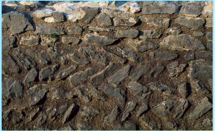
Herringbone masonry was common in castles built by the Normans.
