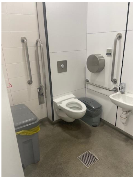
Accessible toilet at Group Admissions
