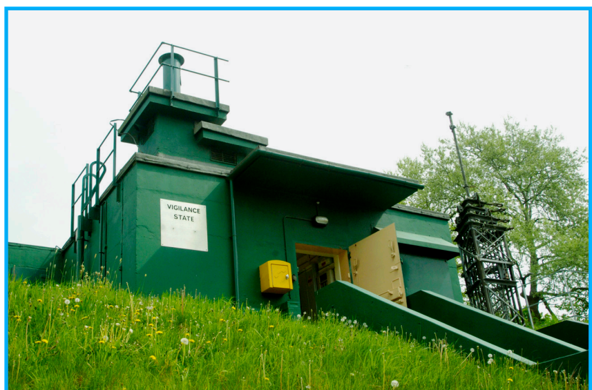
York Cold War Bunker played a key role in nuclear monitoring during the Cold War.
